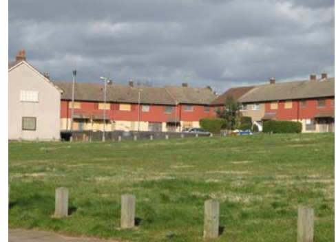
Existing council housing at Wood End
