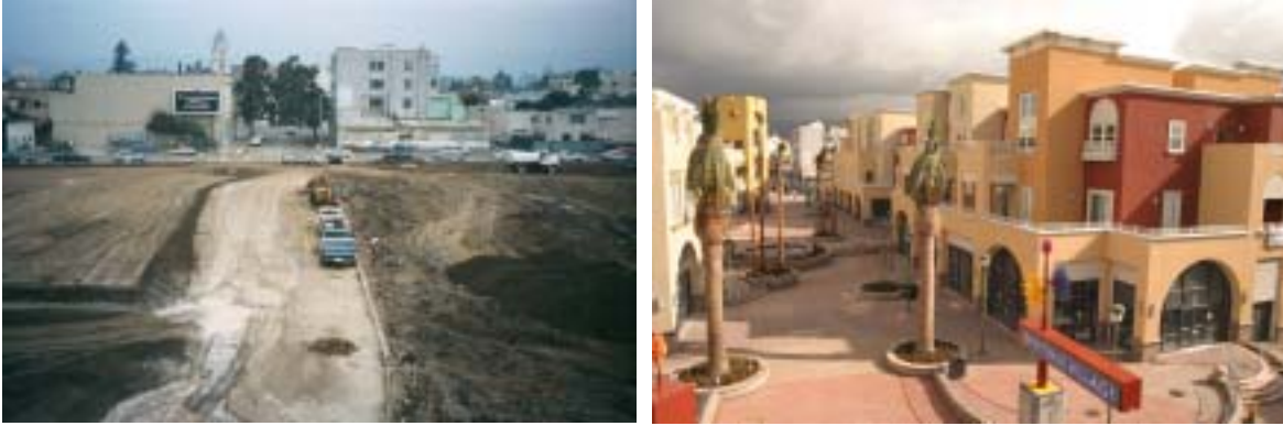
Fruitvale Village from the adjacent BART station. Before (left) and after (right). Photos courtesy of Fruitvale Development Corporation.
