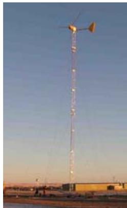
The Liberty County wind turbine is designed to offset electrical power used by the county's maintenance shop, as well as provide a working example of how wind power can benefit local government. The turbine sits atop a 100 ft tilt-up tower and interconnected to Northwestern Energy's distribution grid. The turbine was installed in December of 2003. County Commissioner, Don Marble, championed the installation and currently serves as OWC's Vice President.
