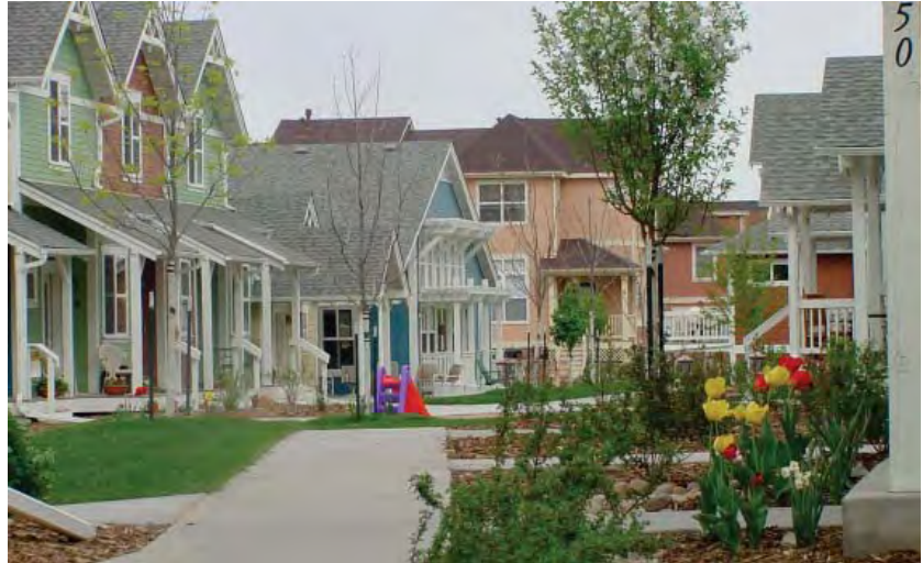
The neighborhood surrounding Highlands Garden Village, a mixed-income, mixed-use urban infill project near downtown Denver, provided significant input on the project design, greatly enhancing its success.
